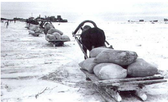
The ice road over frozen Lake Ladoga, "The Road of Life" – tried first on foot, then testing the ice strength on sleds, then with empty trucks, then finally heavily loaded trucks.
