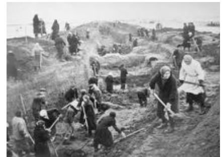
Women dig anti-tank trenches.
